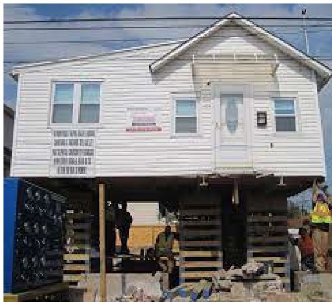
Figure 23: Home in the process of being elevated.
