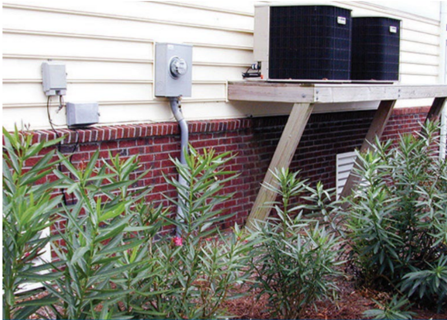
Figure 26: HVAC (Heating, Ventilation, Air Conditioning) unit elevated above base flood elevation.
