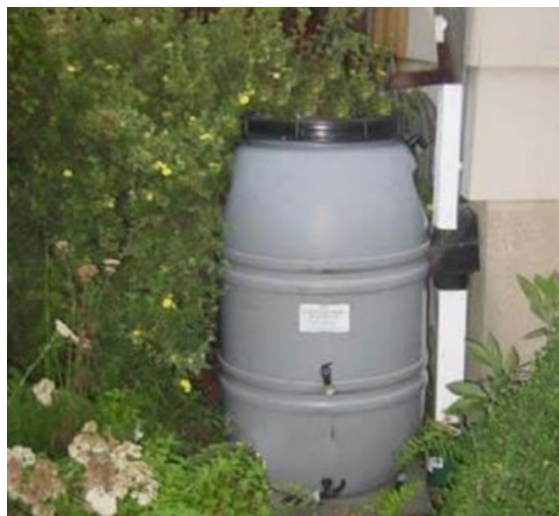
Figure 24: Rain barrels collect stormwater runoff from roofs for reuse.
